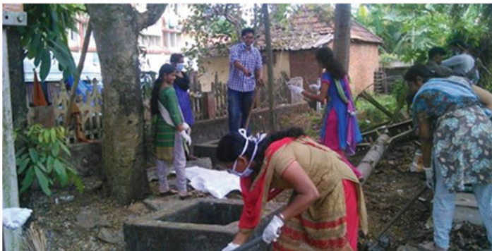
Cleaning Chengannoor Railway Station, and setting up of "Fragrance Garden"
